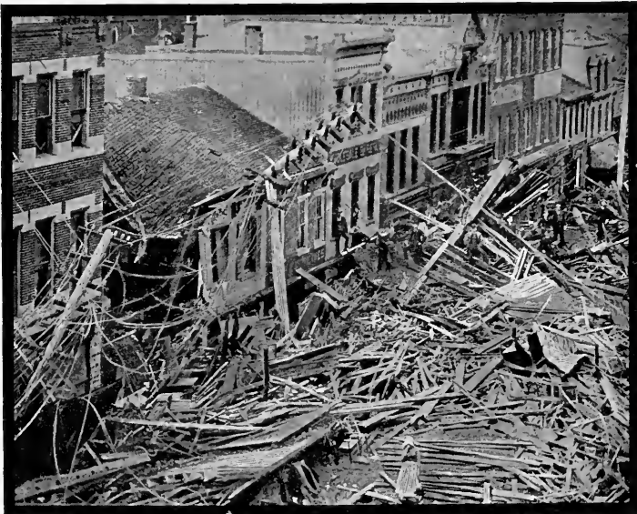
MAIN STREET, JOHNSTOWN, AFTER THE FLOOD
